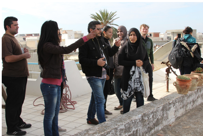
Image: Mounting routers on rooftops.
