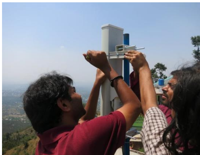
First-time network technicians setting up a long distance link using a Rocket.
