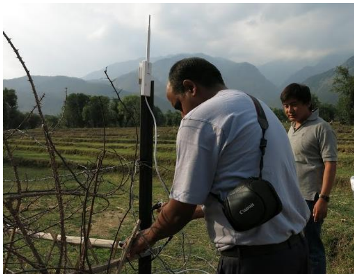
Temporary network installation to test the network reach.
